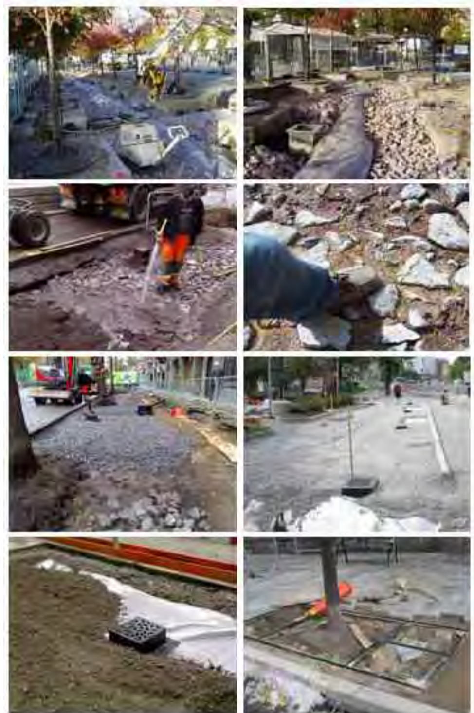
The pictures above illustrate the procedure for structural soil construction, from laying and compressing the crushed rock layers for the structural volume, through protection of existing pipelines, placement of air inlets housing in-planting soil fertilisation, laying aerated bearing layer, laying material-separating geotextile and gravel, placement of drain covers for water gutters to final placement of the tree grid and paving.
